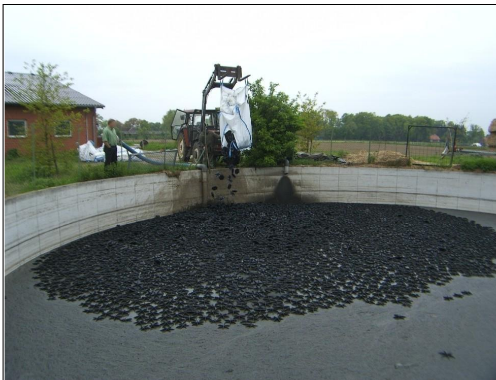
Figure 4.79: Load operation of geometrical plastic tiles into a slurry tank (Hexa-Cover)
