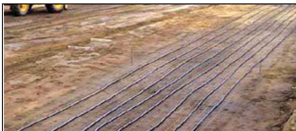
Figure 4.30: Example of PE pipes ready to be cast in concrete
