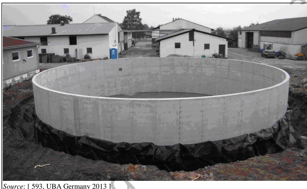
Figure 4.80: Below-ground slurry tank with liquid-tight geomembrane
