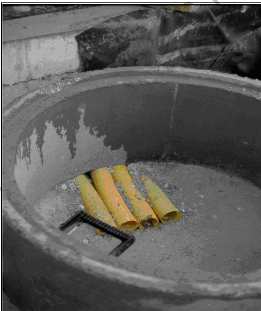
Figure 4.81: Inspection shaft for area drainage pipes from a slurry store
