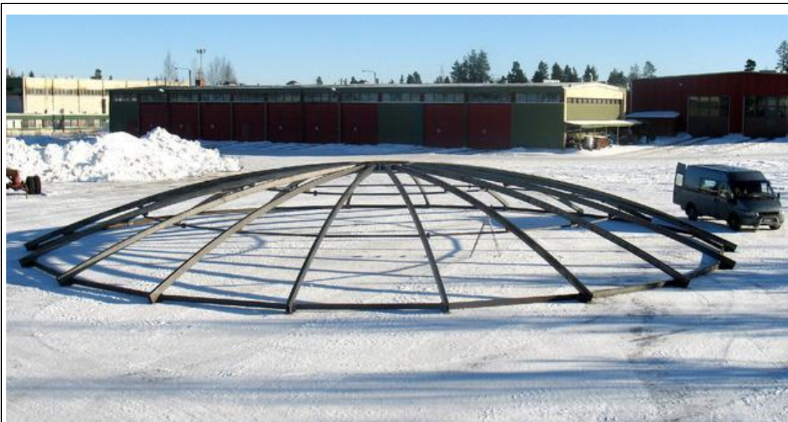
Figure 4.78: Dome-shaped steel structure for a flexible tent before its placement over the slurry store.
